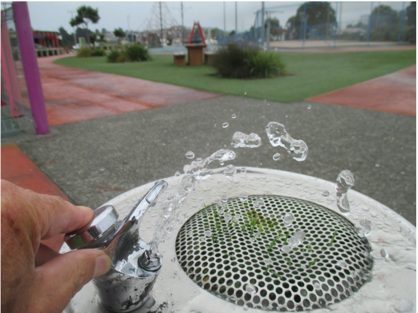
Figure 1: Poorly maintained fountain with grass growing in the drainage sink.
